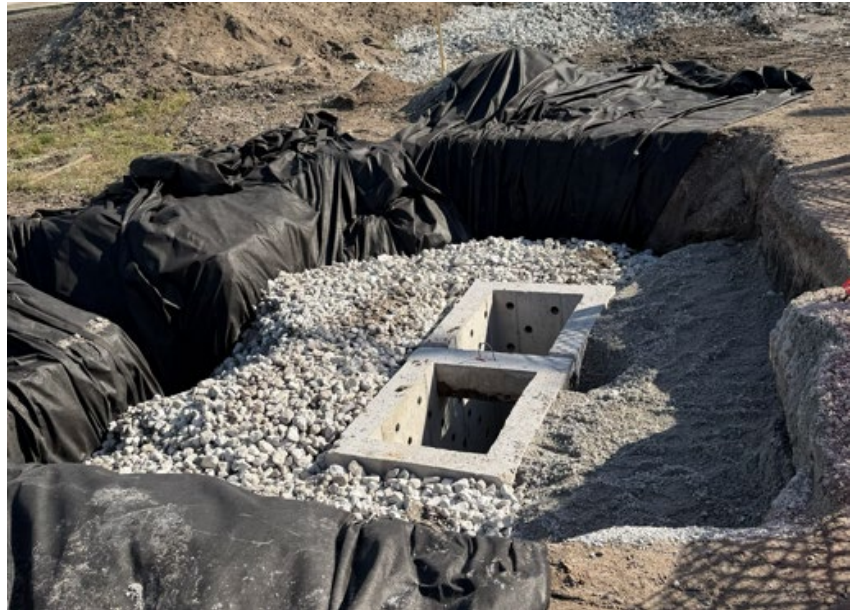
Images of stormwater intake structures and rock infiltration chambers along Freel Drive.
