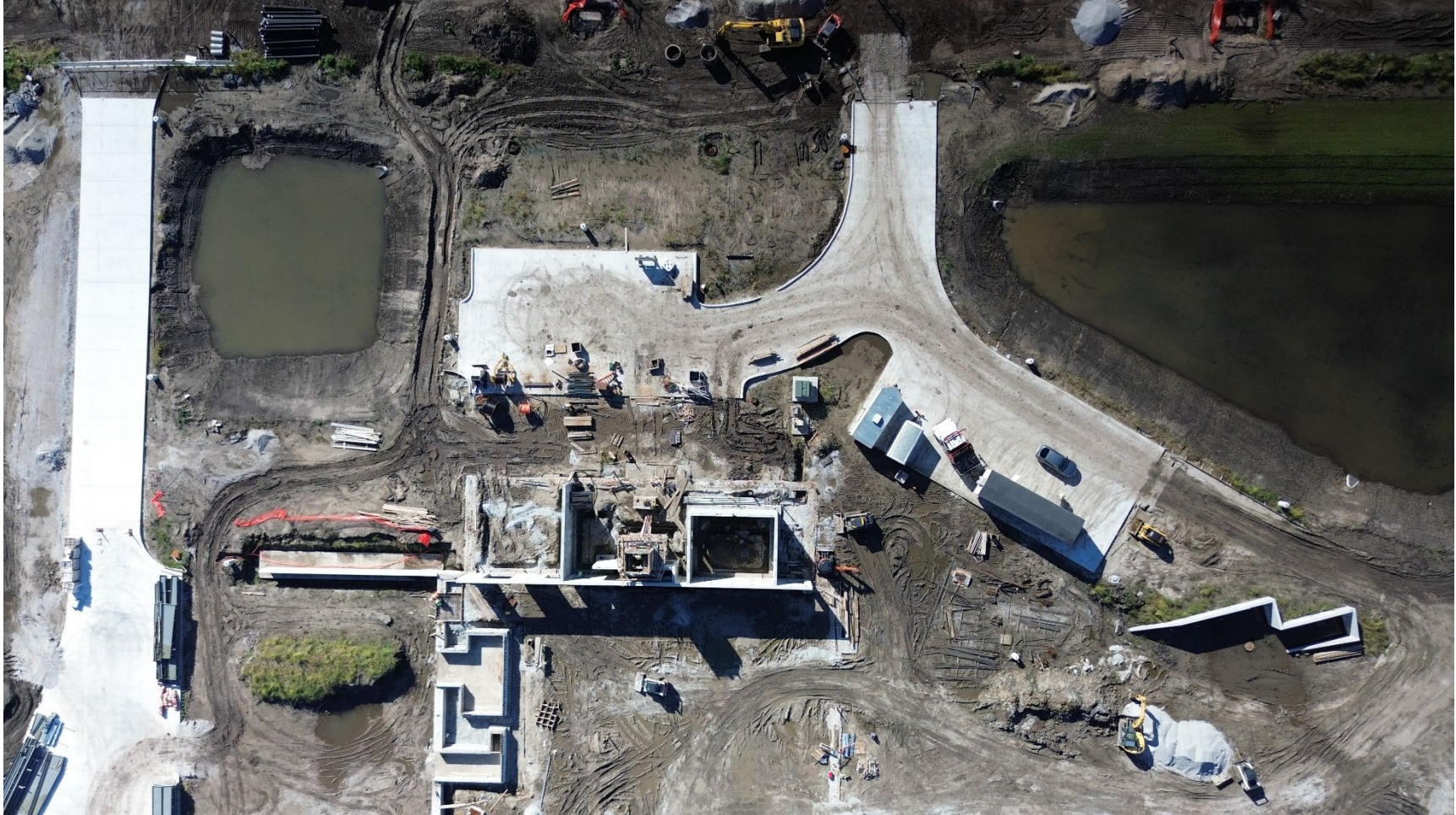
Aerial photo of the R3C site, taken the week of September 30, 2026. At left is a City vehicle entrance driveway. At center is the office area. Equipment and roll-off box pits are to the left of the future tipping floor. The primary shredder will be situated in one pit; the others will contain boxes to collect ferrous and non-ferrous metals that are removed from the solid waste. The customer convenience area is at right, near the detention basin. To its right is the Z-wall, where self-hauled solid waste will be dumped into large rollofs located below. Freel Drive is along the top of the photo. Photo courtesy of Kevin Buck.
