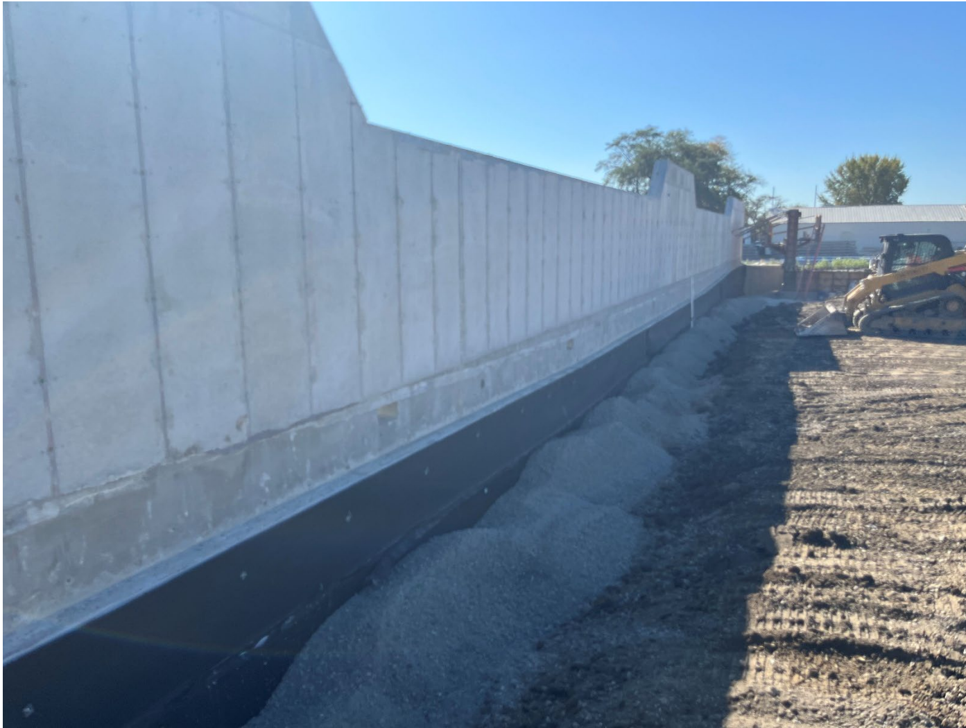
Transfer tunnel wall being backfilled. This area will be paved with concrete containing quartz aggregate to improve abrasion resistance. Looking south-east.
