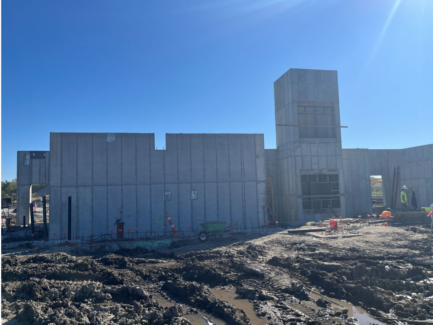
Cast-in-place walls for the locker room and elevator shaft. The locker room will serve as a hardened shelter area in the event of severe weather. Looking east.
