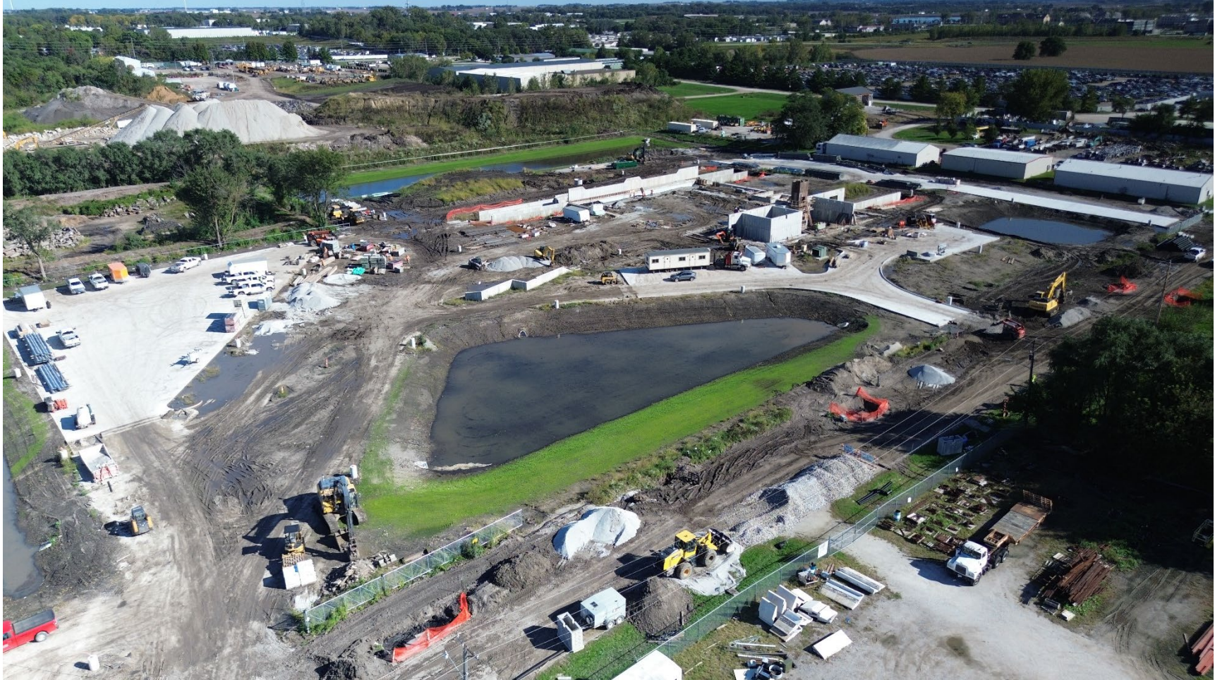
Aerial photo of the R3C site looking east, taken the week of September 30, 2026. The paved area at left is the truck and trailer parking area. At center, where a job trailer is parked, is the future customer convenience area. To the right is the office area of the building. At the rear is the transfer tunnel. Freel Drive is running diagonally near the bottom of the photo. Photo courtesy of Kevin Buck.
