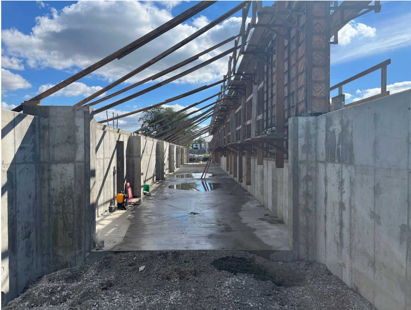
Looking south through the transfer tunnel.
