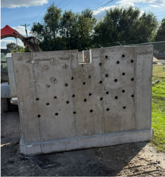
Images of stormwater intake structures and rock infiltration chambers along Freel Drive.
