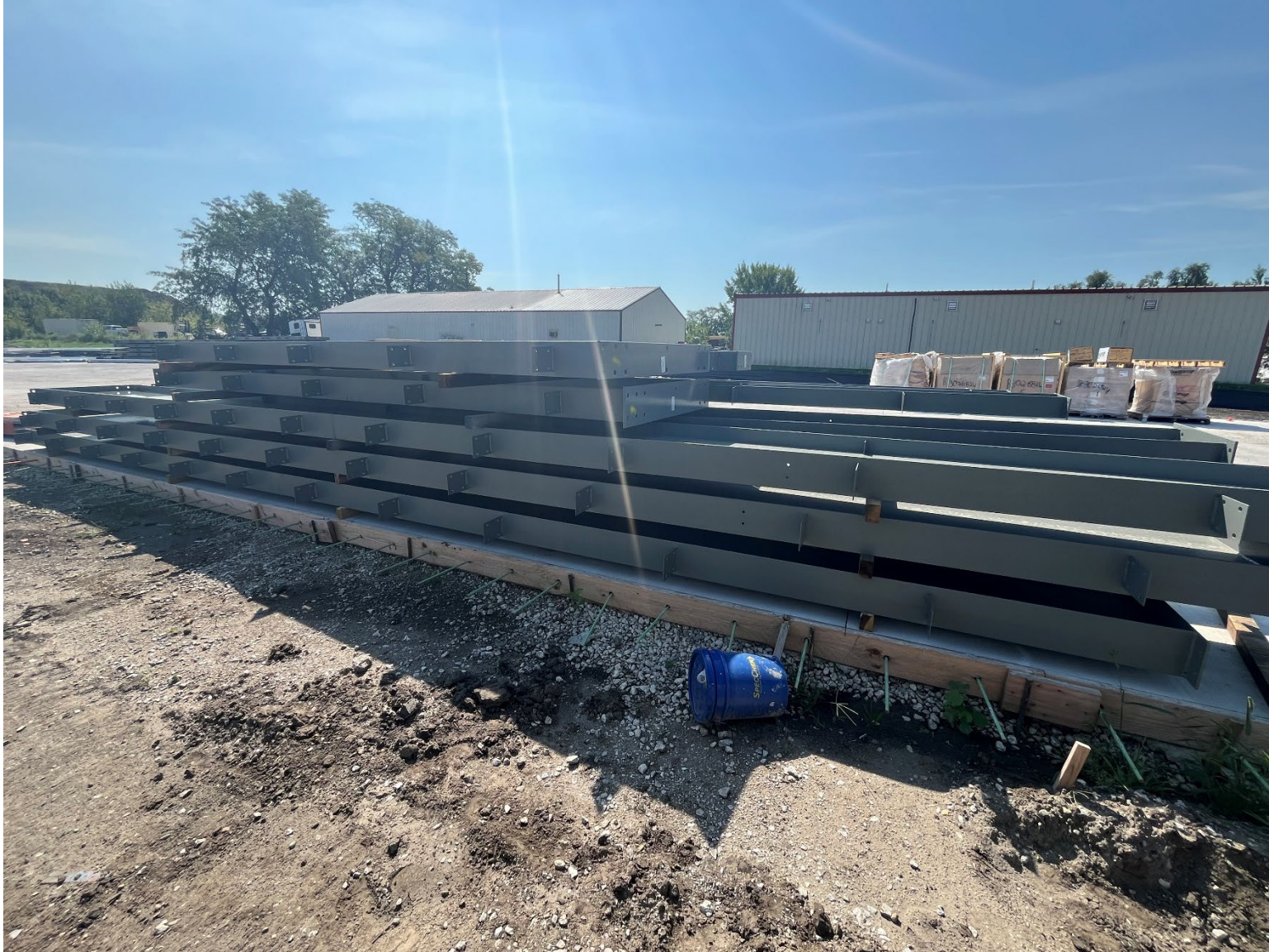
Structural steel for the pre-engineered metal building. Building erection begins this month.
