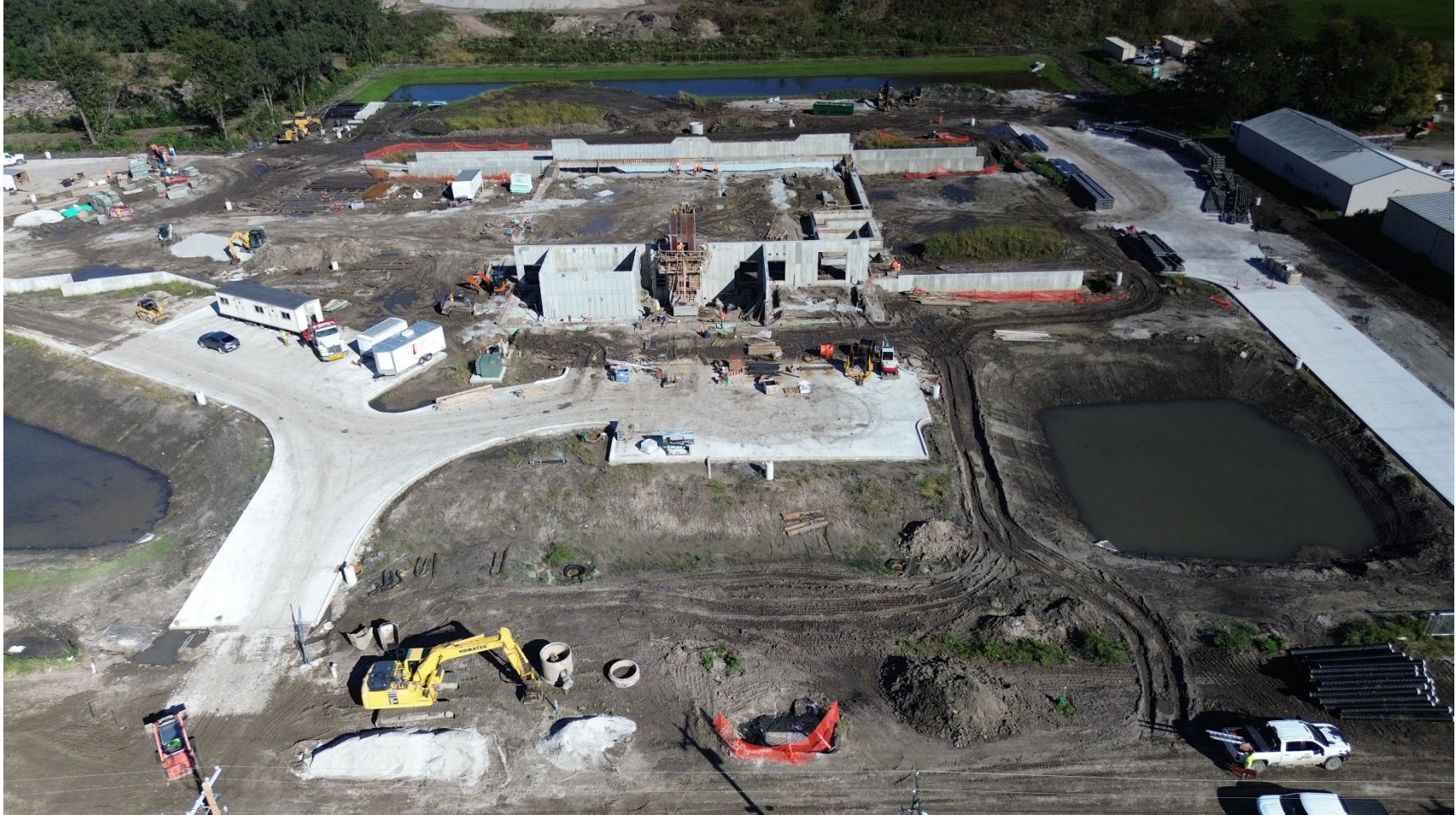
Aerial photo of the R3C site looking east, taken the week of September 30, 2026. Centered is the office parking lot, with the office behind. At the rear is the transfer tunnel. Freel Drive is running along the bottom of the photo. Photo courtesy of Kevin Buck.
