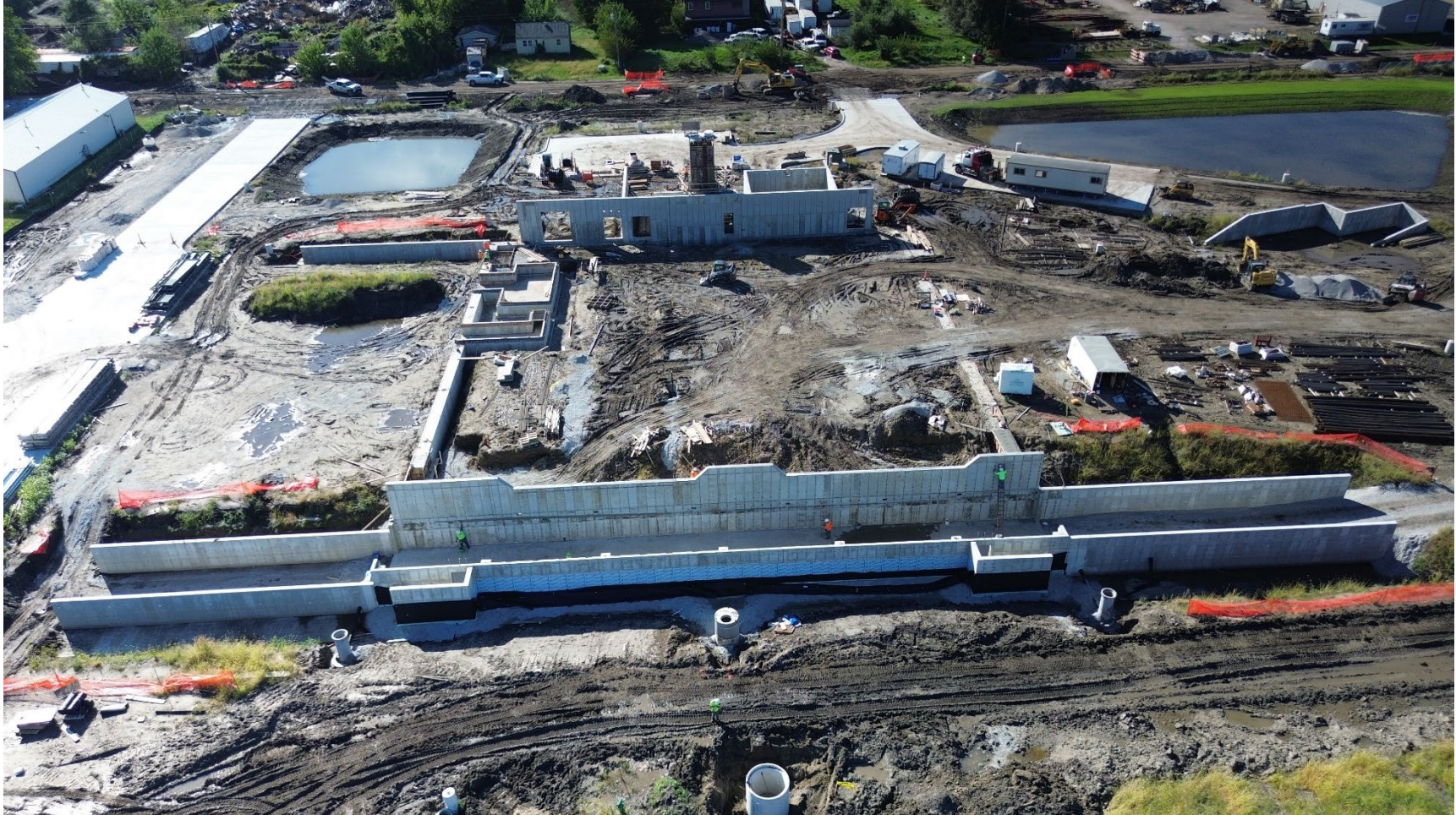
Aerial photo of the R3C site looking west, taken the week of September 30, 2026. The transfer tunnel is at the bottom of the photo. Trucks will enter from the left, be loaded in the center, and will exit up the ramp at right. The office area is at the back of the photo. In between is the future tipping floor space. Openings at the right will allow commercial haulers to enter and exit the tipping floor. Freel Drive is along the top of the photo. Photo courtesy of Kevin Buck.
