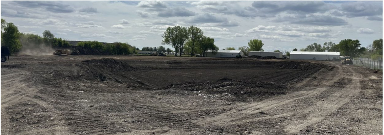
R3C Earthwork Overview
