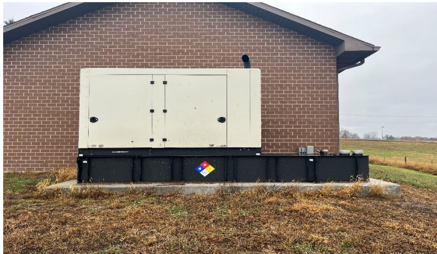
New standby generator installed at the SAM Pump Station
