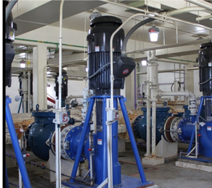
Trickling Filter Pumps
