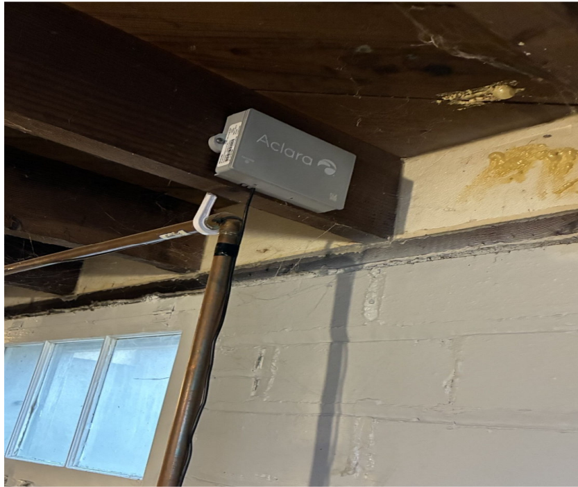
Aclara Meter Transmitter Unit (MTU) mounted on the floor joist in the basement of an Ames resident's home
