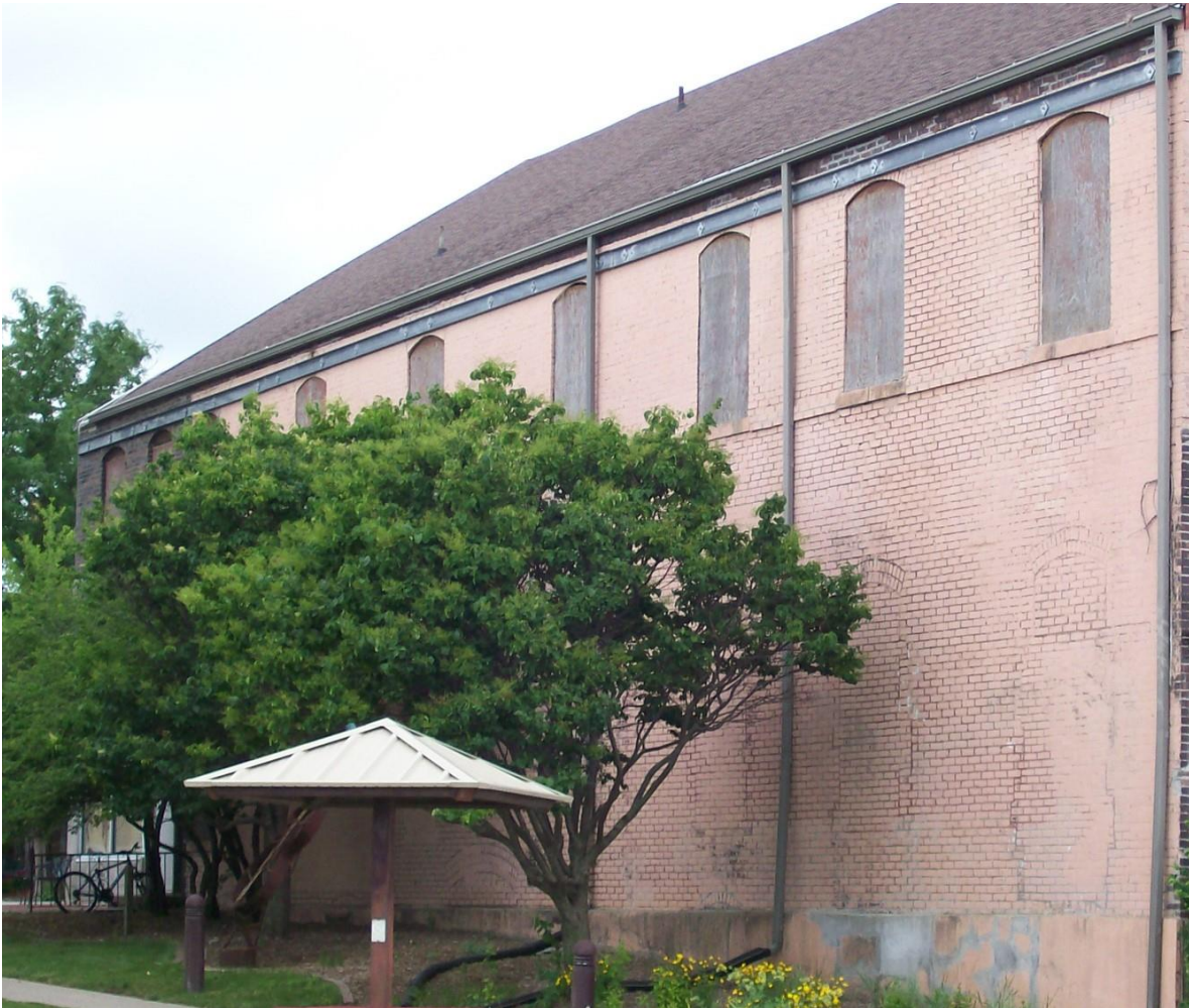
Existing Façade for 330 Main Street
