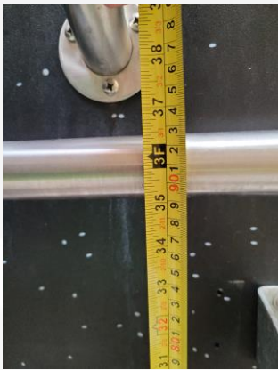
Grab bars located outside of compliant range
