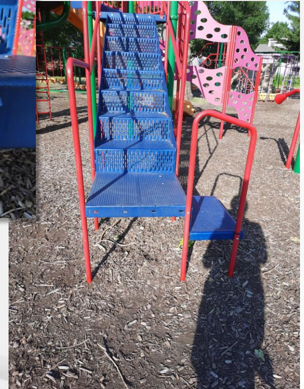
Transfer platform too high
