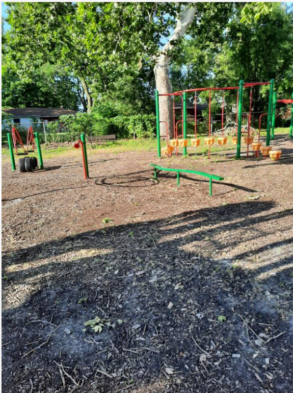
Surface in disrepair
