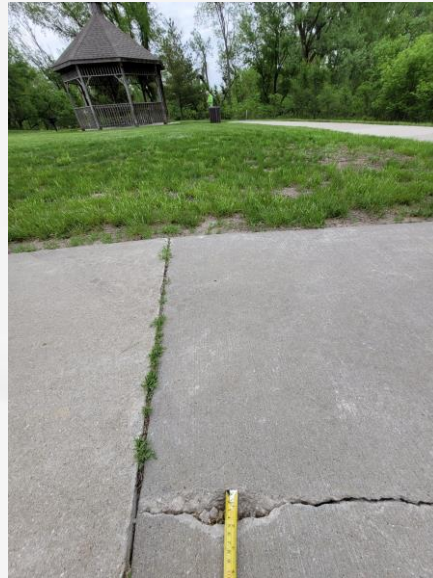
Surface deterioration along path
