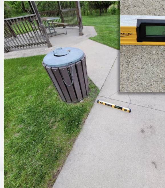
Cross slope of clear floor space exceeds 2.08%
