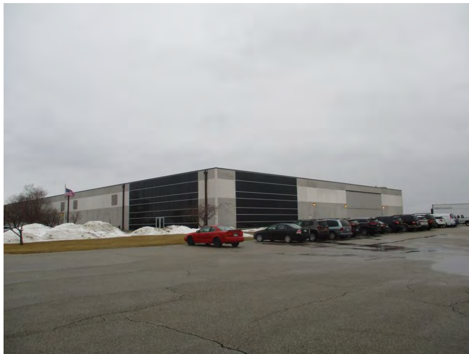
Southeast Building Elevation - Warehouse
