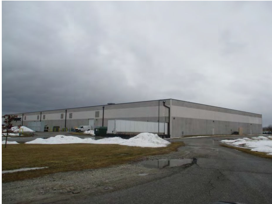
Northwest Building Elevation - Warehouse
