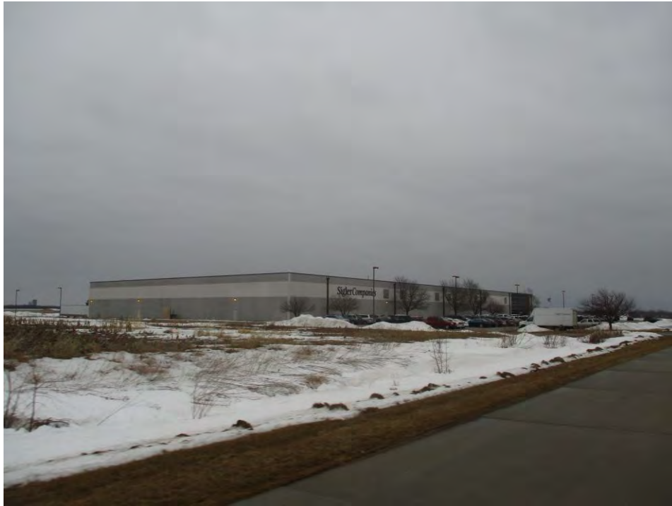
Looking Northeast at Subject Property
