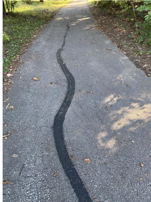
Asphalt Crack Filling/ Joint Repair Examples
