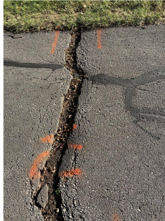
Asphalt Crack Filling/ Joint Repair Examples
