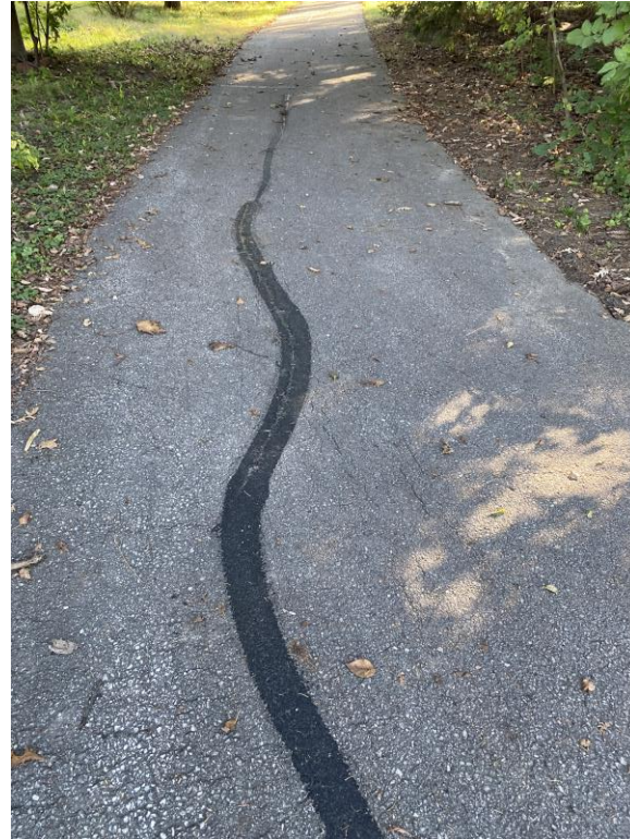
Asphalt Crack Filling/ Joint Repair Examples
