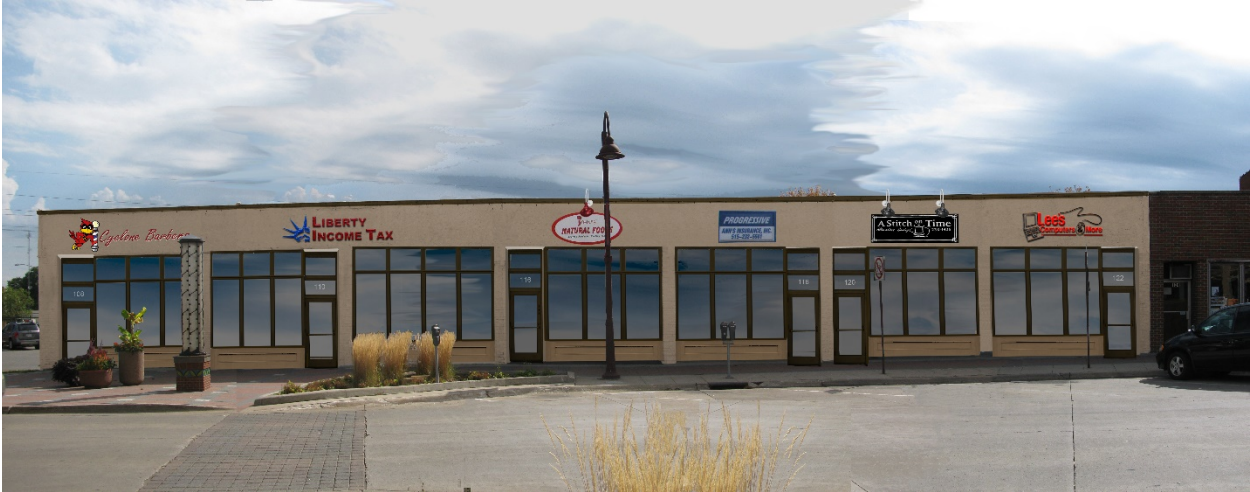
Proposed Final Façade (108 Main Street is the storeront on the left)
