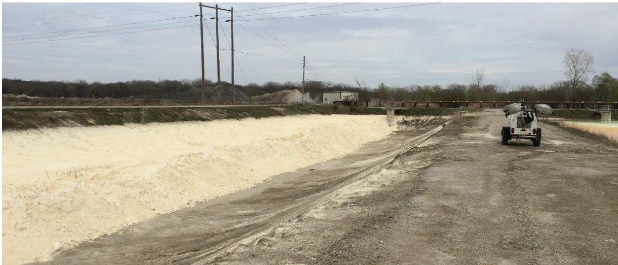
A lime pond cell after having one half of the contents excavated.
