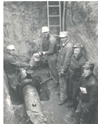
Water main break repair in Ames Circa 1953
