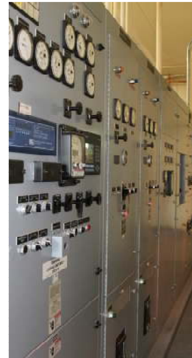
Cogeneration switchgear Ames Water Pollution Control Facility
