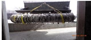
Primary shredder rotor replacement
