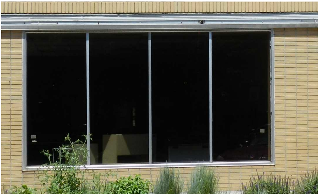
#08: EXISTING ALUMINUM WINDOWS Iowa Electric Light & Power Company 131 Main Street Ames, Iowa August 26, 2017
