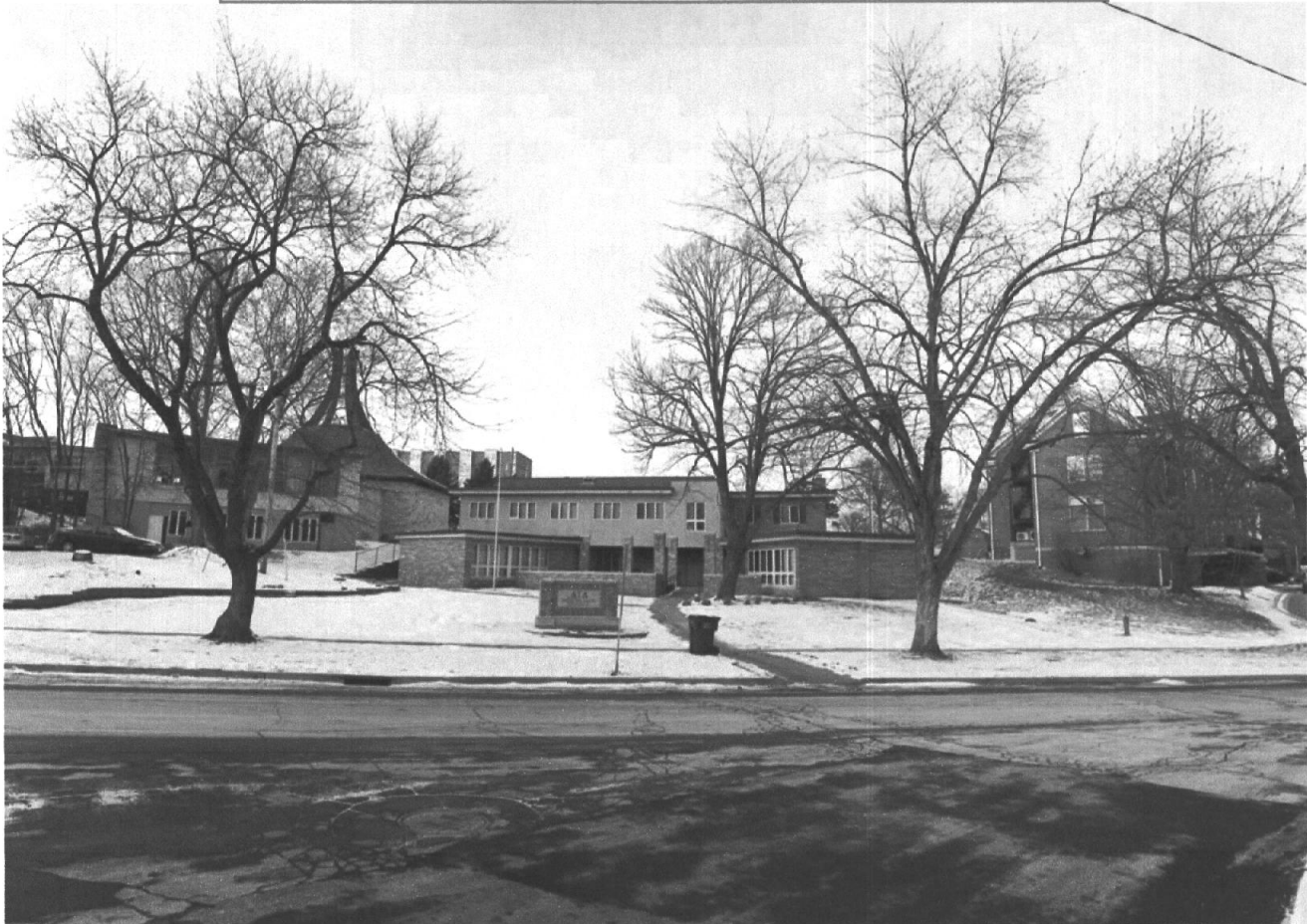
Current Delta Tau Delta building (view to north from Sunset Drive)
