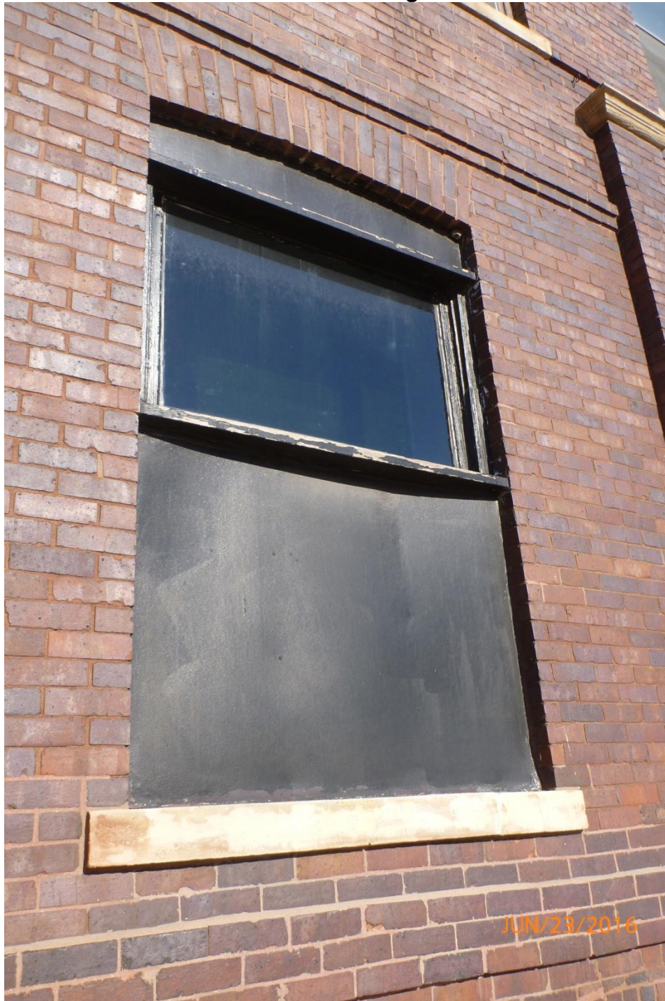
First Floor Window
