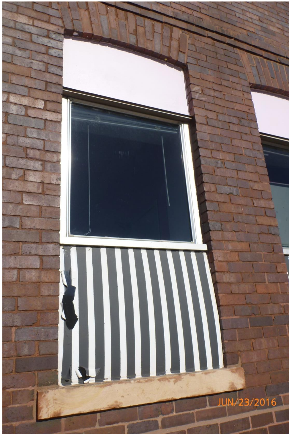
First Floor Window
