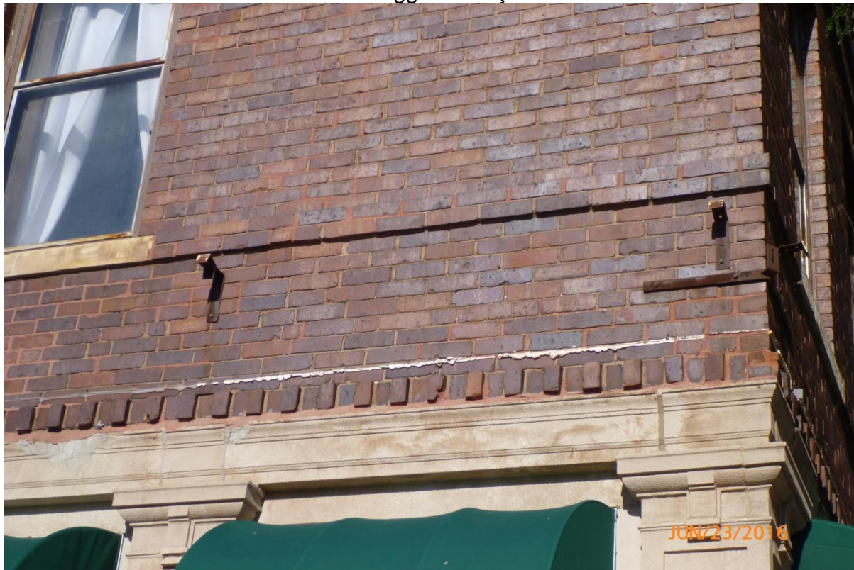
Old Fasteners to be Removed (2 of many)
