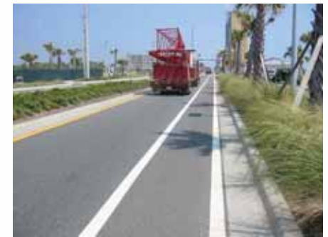
This road in Panama City Beach, FL has 10-foot lanes (which easily accommodate large trucks) adjacent to 5-foot designated bike lanes (4 feet of asphalt, plus gutter pan).
