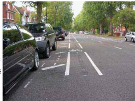
(Top) An example of a bike lane located within the “door zone” of the adjacent parallel parking lane. (Bottom) Providing a striped buffer between on-street parking and a bicycle lane is a potential design solution to encourage riding outside the “door zone”.
