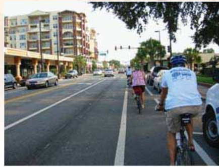
A “road diet” project converted Edgewater Drive in Orlando, FL from a 4-lane undivided roadway to 2-lanes with center turn lane and bicycle lanes.
