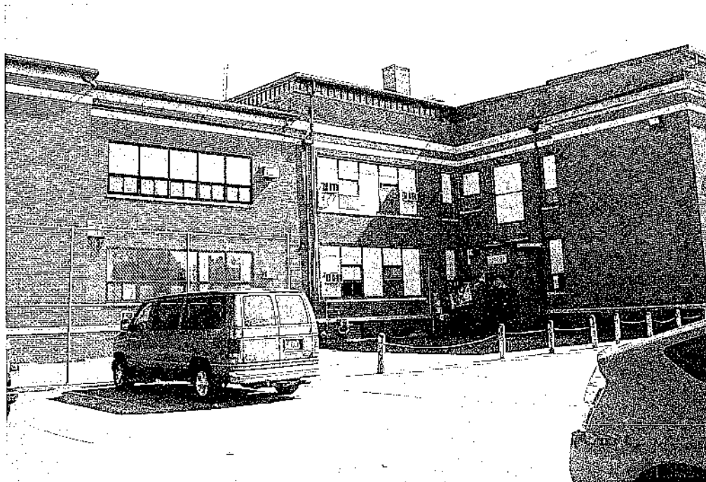
Rear of original Roosevelt School building, View to the SE with 1968 gymnasium addition to left
