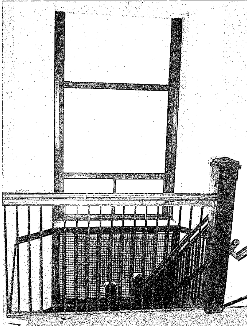
Interior stairwell of original Roosevelt School building showing original woodwork and metal and wood stair rails
