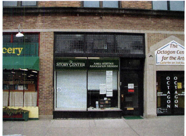
Transom windows at 417 Douglas Avenue—a good historic design carefully maintained.
