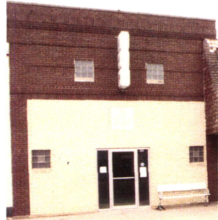
An inappropriate storefront treatment.
