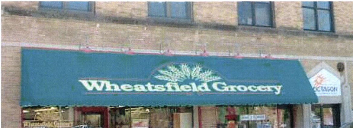
Fabric awnings with loose valences and triangular frame. Two options for signs on awning are shown.
