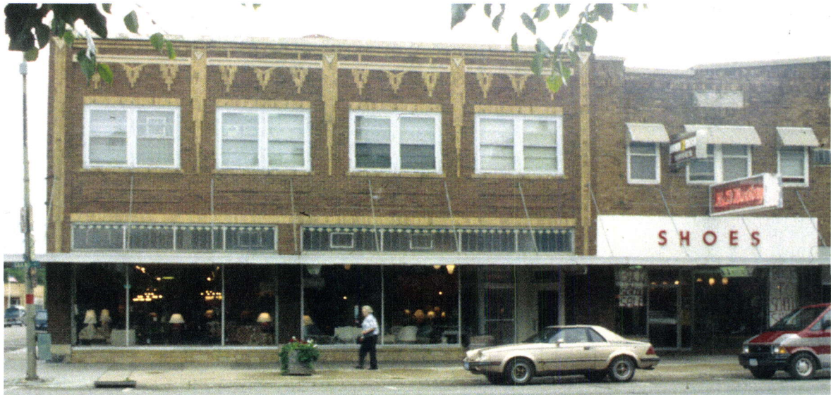
Two transom treatments in Spencer, Iowa. The building at left retains its original transoms. (A flat canopy was installed at a later time.) The building at the right has masked its transoms. Which building is more appealing? Both buildings need to improve their signage. Perhaps the “Christensen Jewelry” sign technique, (see “Awnings and Canopies” below) would be a good solution for both.
