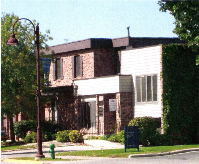
Variation in roof height of more than five feet and flat roof hidden by parapet.
