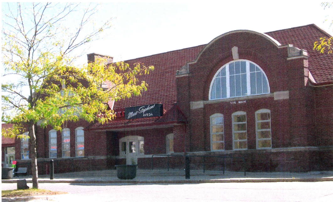
Ames depot building with roof slope steeper than 6:12
