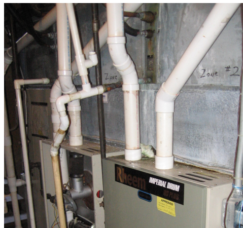
Condensing units and furnaces serving original building NW areas.
