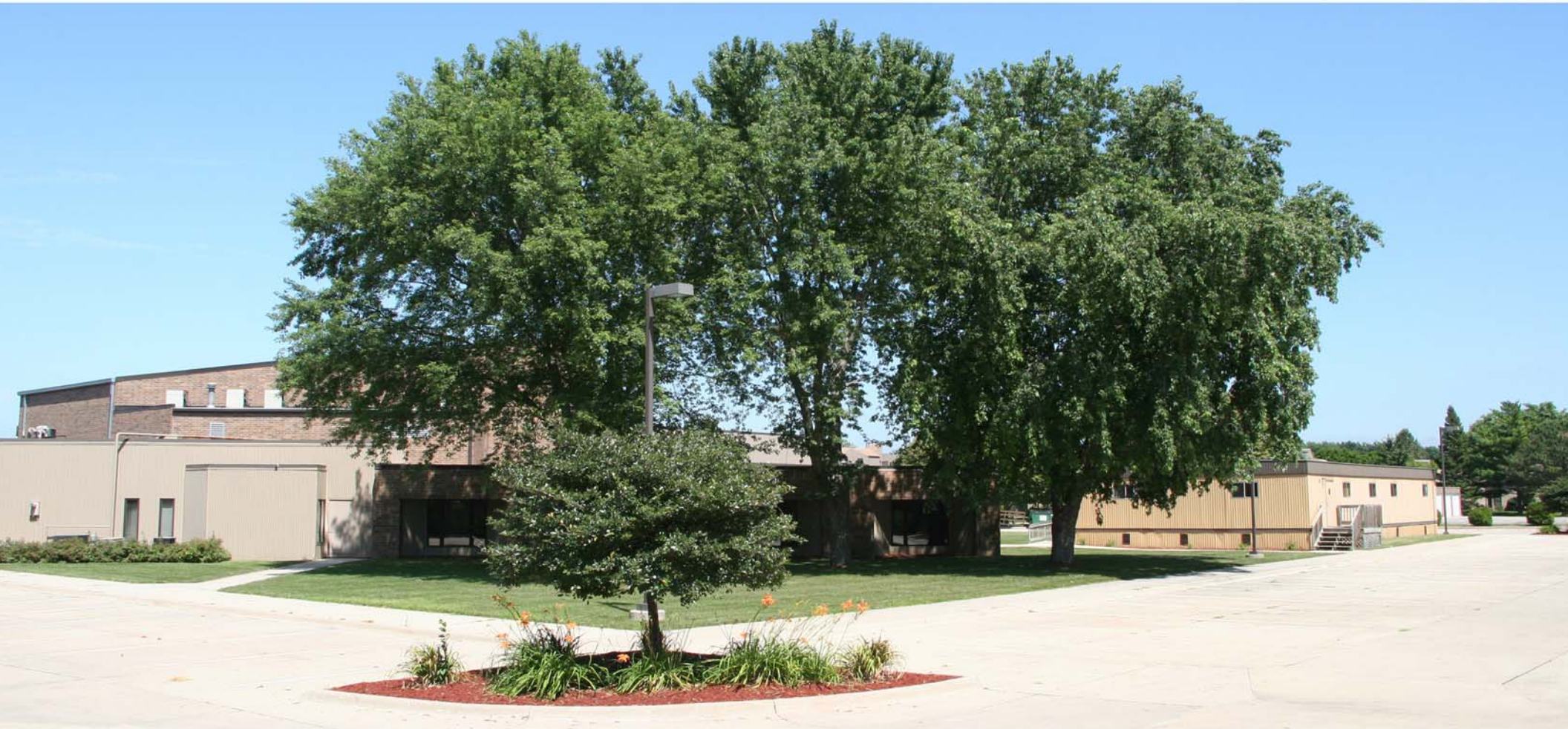
VIEW FROM SOUTHWEST - EXISTING
