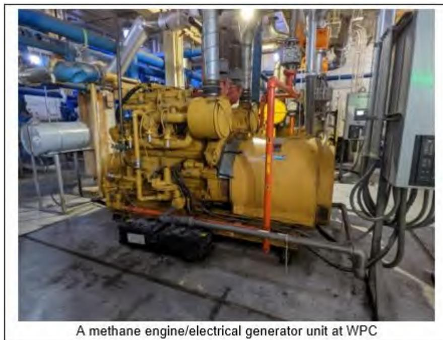
A methane engine/electrical generator unit at WPC
