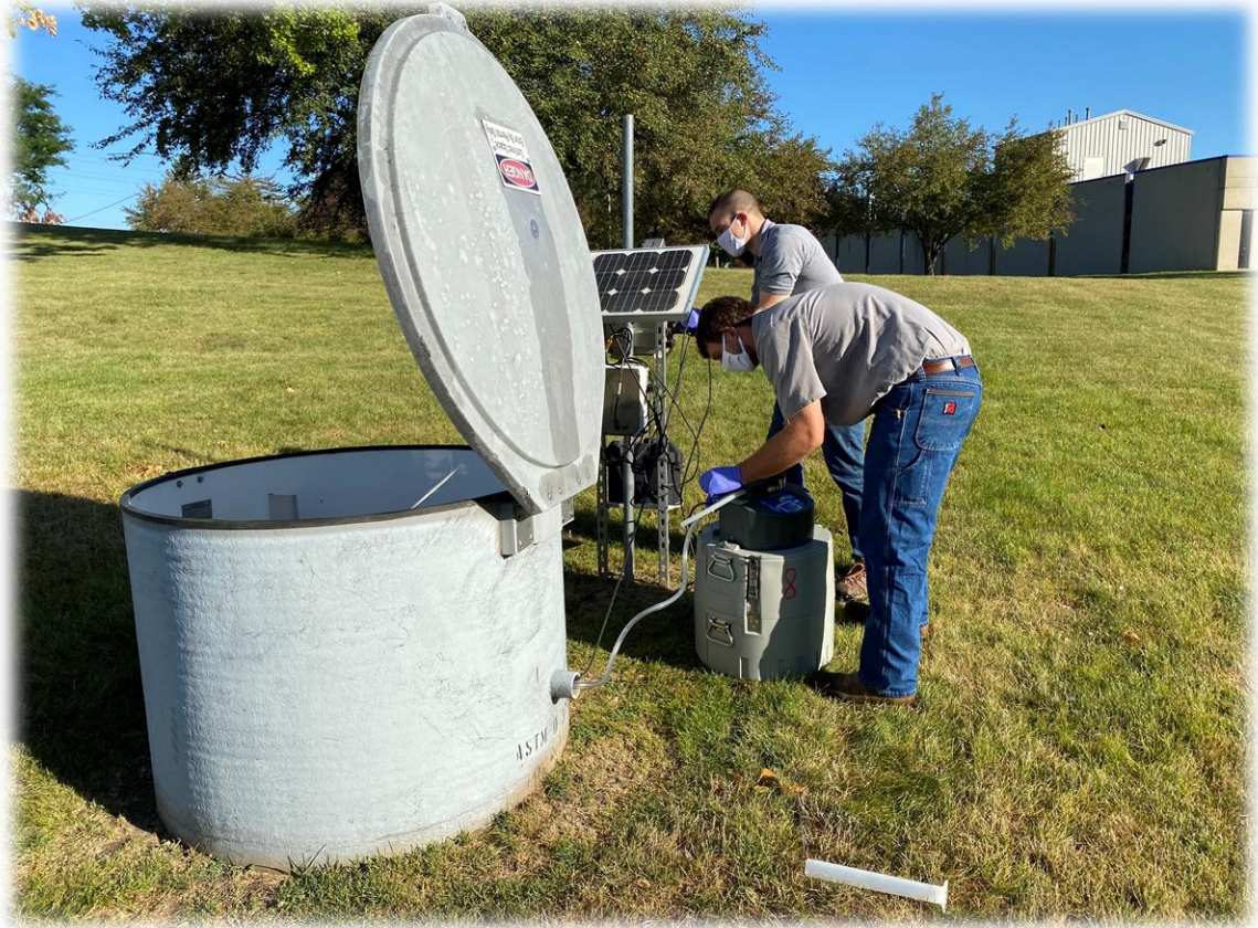
Industrial pretreatment sampling being performed by staff from the Laboratory Services and WPC Facility Divisions
