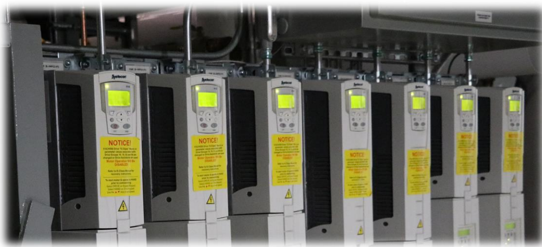
Boiler controls at the new Water Plant
