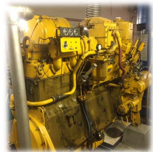
Diesel engine at Old High Service Pump Station
