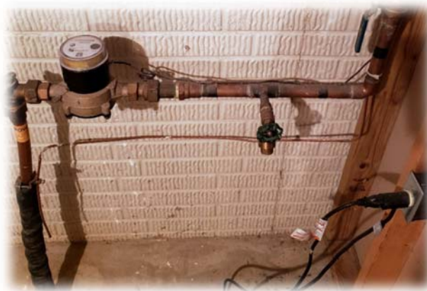
A typical residential water meter installation
