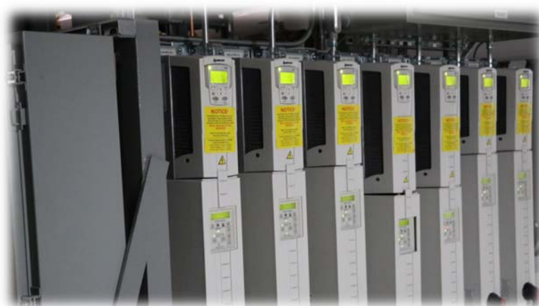
Boiler controls at the new Water Plant
