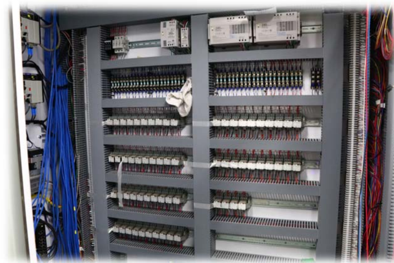
Control panel during construction
