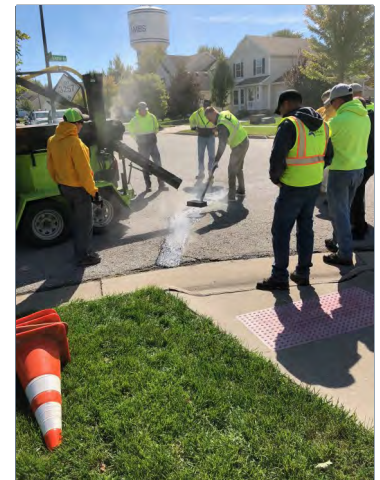
Operations Staff training on the process to use mastic to fill deep cracks on streets and share use paths
