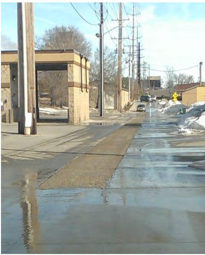
Photo 1: Pervious concrete on Gilchrist Street to improve water quality in S. Skunk River basin.
