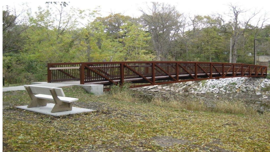
Brookside Park Bridge - Finished
