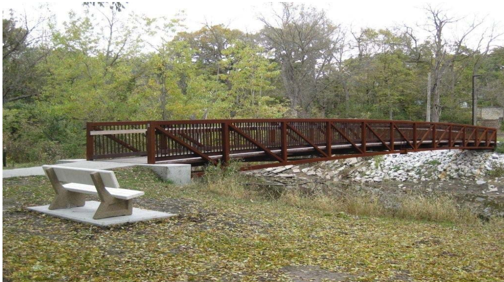
Brookside Park Bridge - Finished
