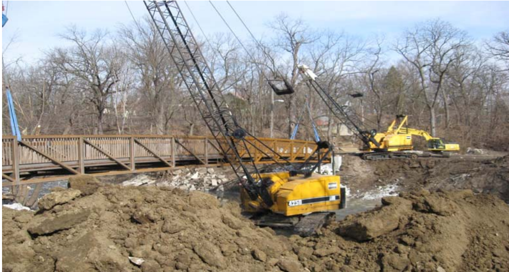
Brookside Park Bridge – Under Construction
