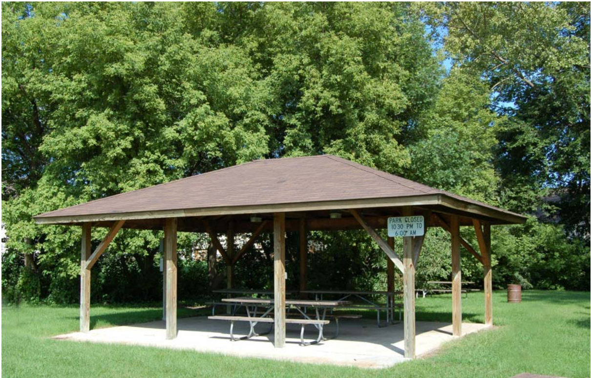
In 1997, the neighbors of Country Gables Park constructed an 18-ft. x 24 ft. open shelter, using Neighborhood Improvement Program funds as a match to their volunteer labor.
