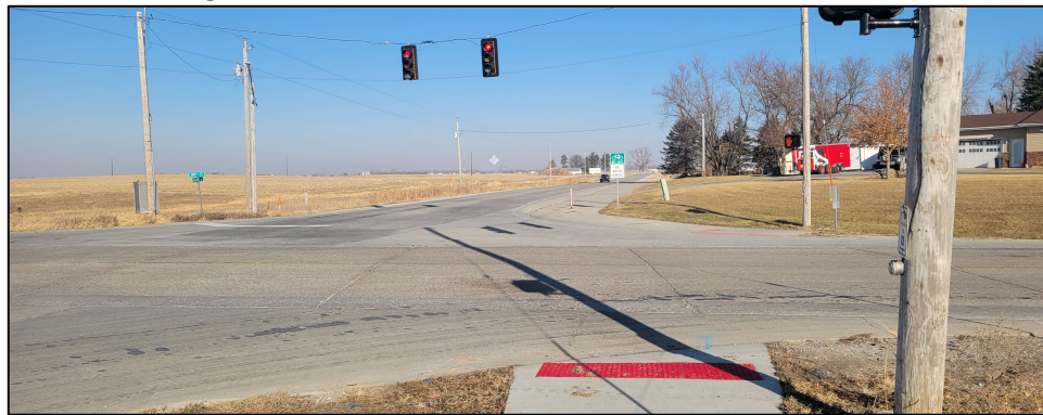
Figure 13 – Grant Avenue Bike Path at W 190 th Street
