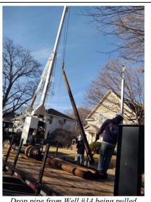
Drop pipe from Well #14 being pulled during rehabilitation on January 6, 2023.
