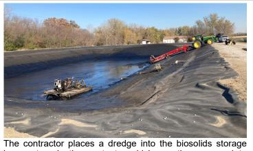
lagoon to mix the contents, which are then pumped to injection equipment in the City-owned farm fields. In the above photo, the lagoon is nearly empty.
