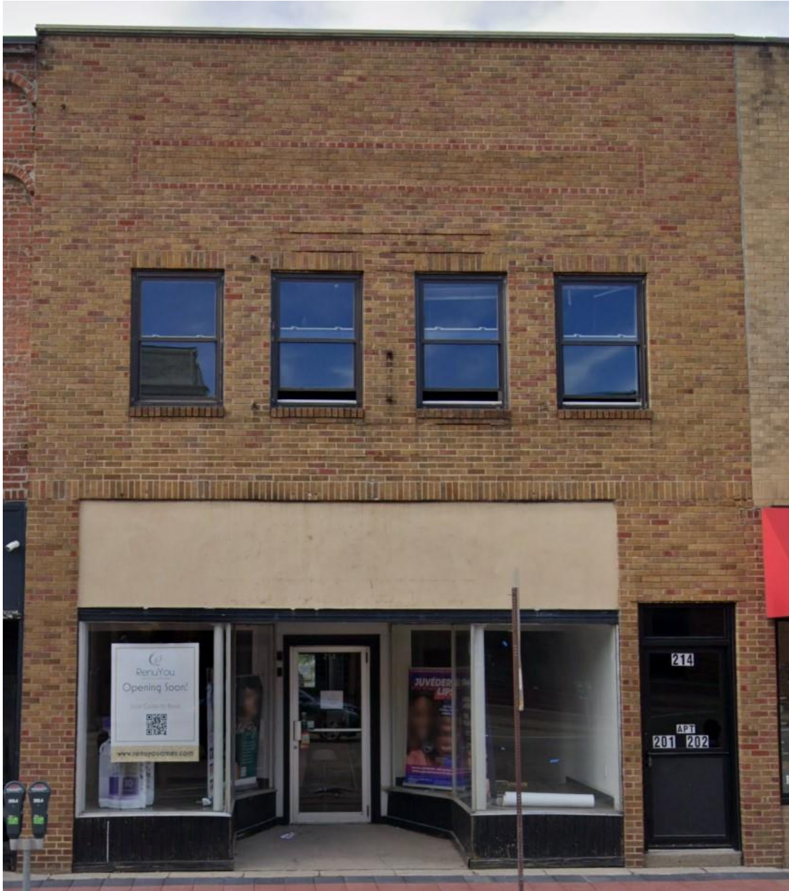
Current Façade for 214 Main Street
