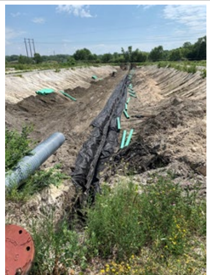
Lime pond underdrain piping staged in advance of installation – August 2, 2021
