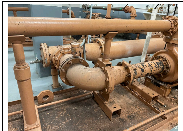
Representative example of the pumps, piping, valves, and paint coatings that will be replaced by this project.
