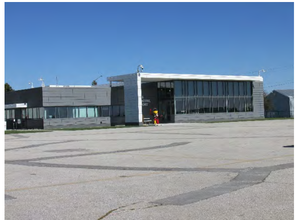
Airport Terminal Building
