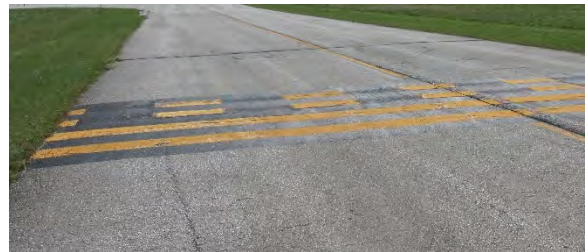
Hold Position Marking
