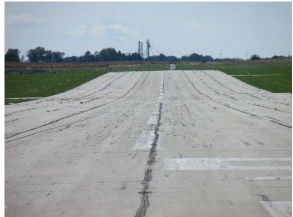
Runway 19 (southwesterly view)
