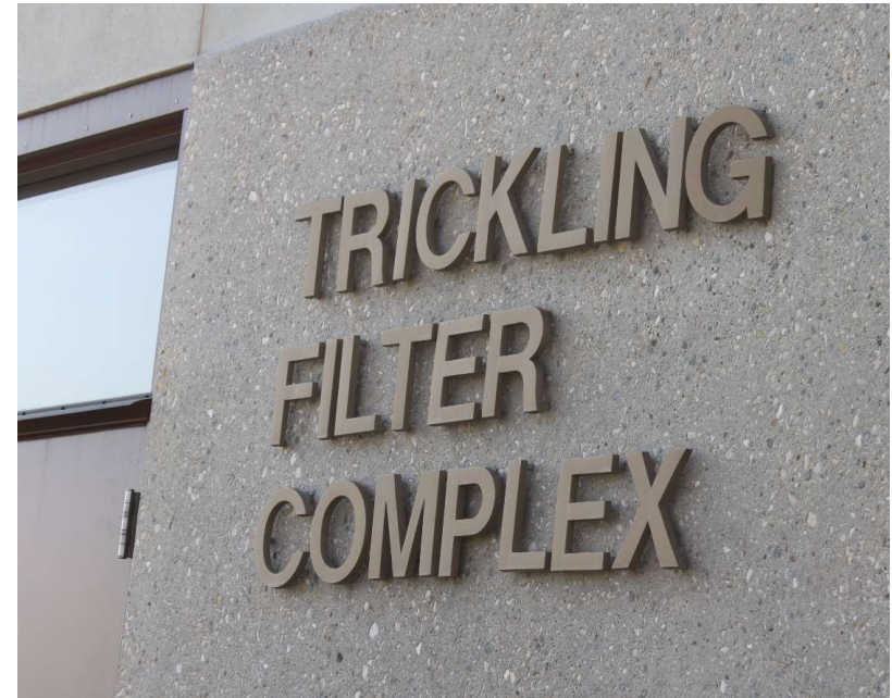
Entry sign into the Trickling Filter Pump Station Ames Water Pollution Control Facility
