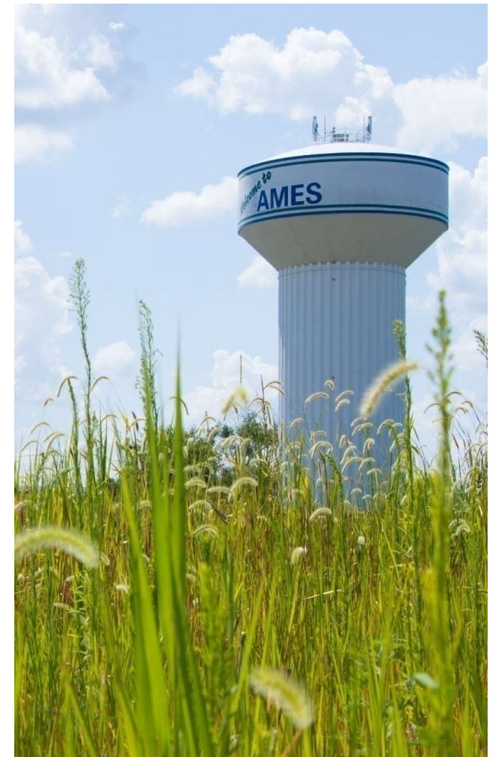
1 million gallon elevated tank Mortensen Road and County Line Road
