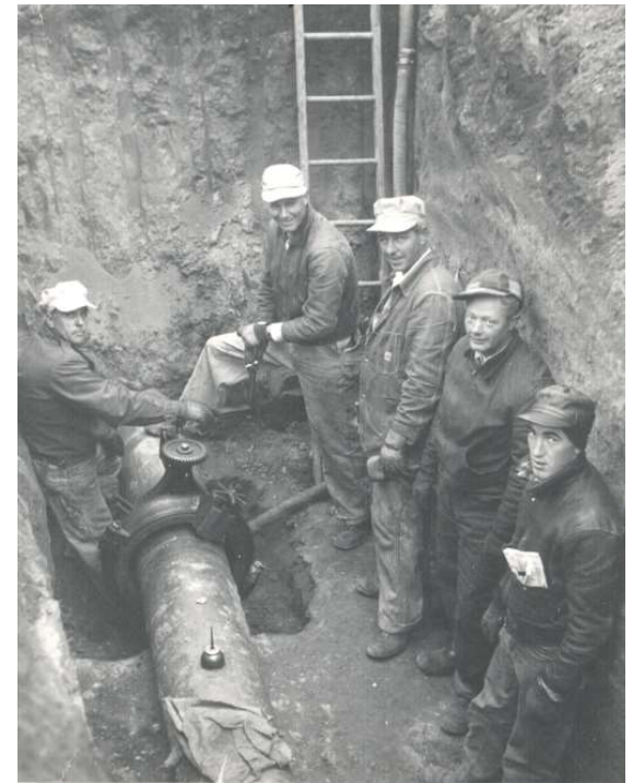
Water main break repair in Ames circa 1953
