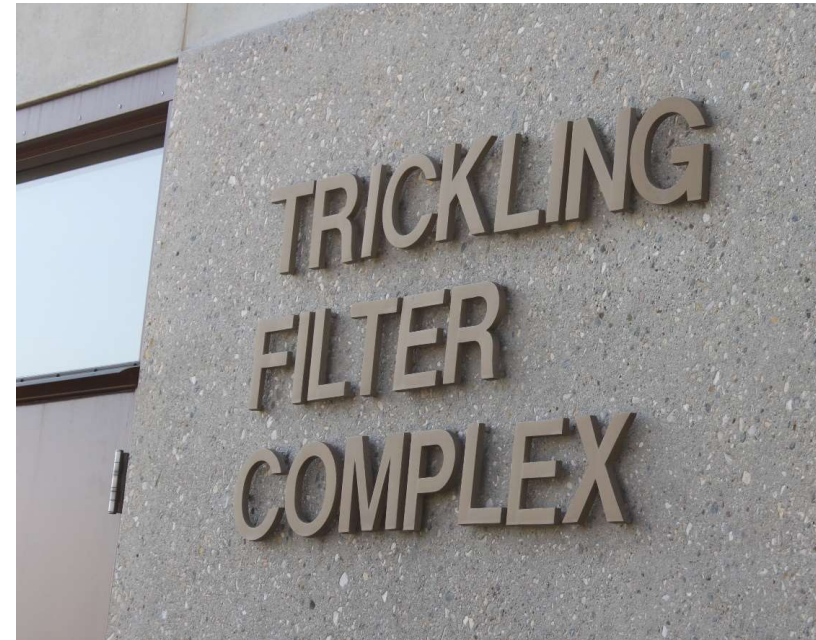
Entry sign into the Trickling Filter Pump Station Ames Water Pollution Control Facility
