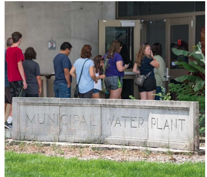
Limestone sign salvaged from the 1924 water plant, relocated to the new facility
