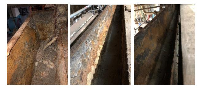
Helfrich will supply and install a new, 304 stainless steel water seal trough, 316 stainless steel saw tooth wear plate, 309 stainless steel baffle, scallop tube, air seals with gaskets and hardware, and W8 and C11 stiffeners. The replacement will involve removing and replacing a 2-foot band of 9-inch thick refractory around the entire perimeter of the bottom ash hopper.
