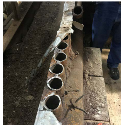
Figure 5 Lower Wall North Side Header
