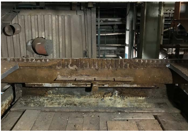
Figure 4 Unit 7 Lower Wall North Side Header
