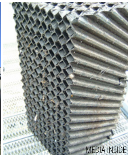
EXISTING TRICKLING FILTERS
