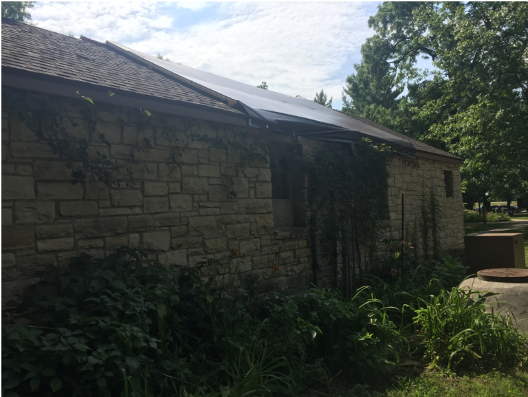
Photo 4 – Exterior masonry in good condition (IMG 6947)
