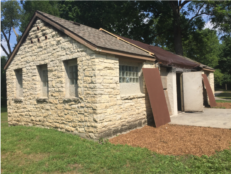
Photo 3 – Exterior masonry in good condition with some smoke and soot discoloration (IMG 6954)
