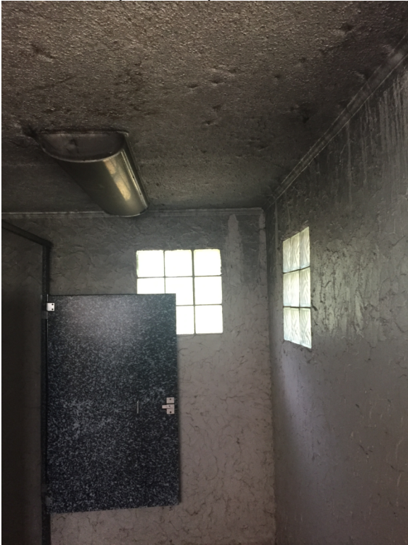
Photo 7 – Interior masonry with stucco surface in good condition with some smoke and soot discoloration (IMG 6931)
