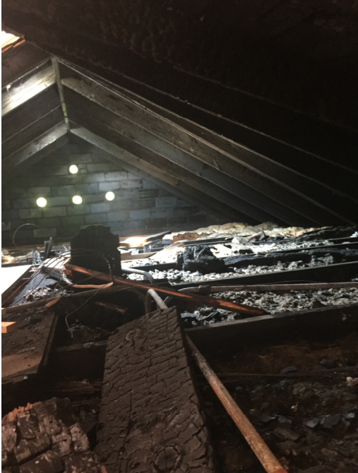
Photo 9 - Any remaining wood roof structure is in poor condition and should be demolished (IMG 6973)
