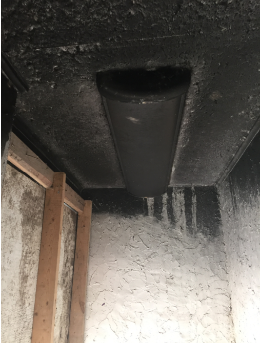
Photo 6 - Interior masonry with stucco surface in good condition with some smoke and soot discoloration (IMG 6935)
