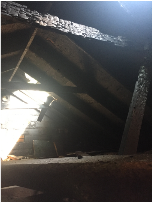
Photo 10 - Any remaining wood roof structure is in poor condition and should be demolished (IMG 6968)
