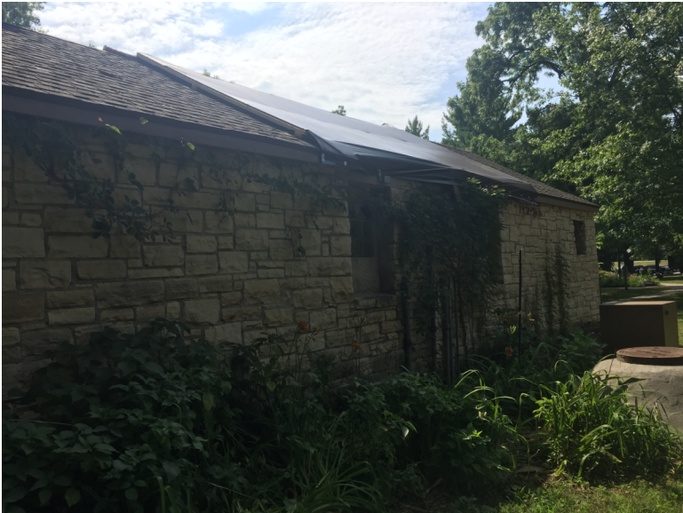
Photo 4 – Exterior masonry in good condition (IMG 6947)
