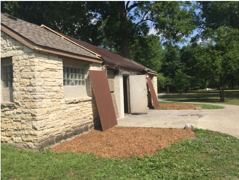
Photo 2 - Front of bathroom structure with canopy and half of roof missing (IMG 6955)
