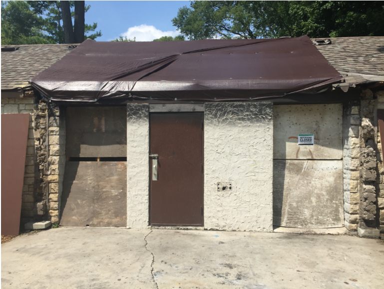
Photo 2 - Front of bathroom structure with canopy and half of roof missing (IMG 6955)
