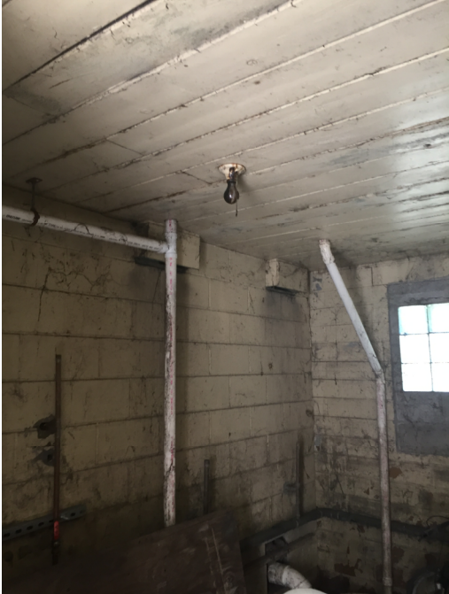
Photo 8 – Interior masonry in good condition (IMG 6958)
