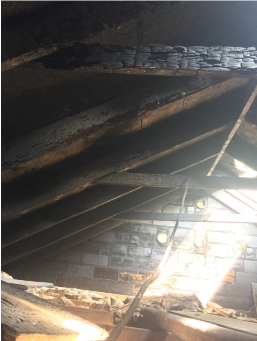
Photo 11 - Any remaining wood roof structure is in poor condition and should be demolished (IMG 6967)
