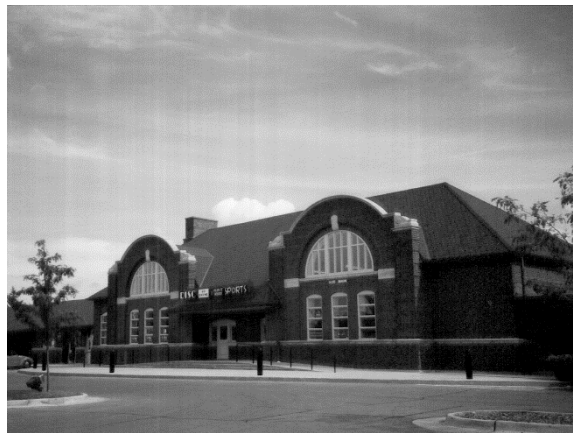
Depot reuse for commercial activities in Downtown Ames
