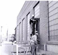
Figure 3: 1956: Walk-Up Teller Window retrofitted into existing glass block opening
