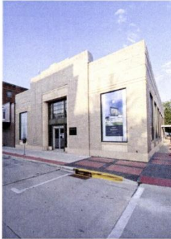
Figure 1: 413 Main Street "Executive Office Building" Primary East Facade
