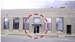
Figure 2: 413 Main Street Secondary North Facade Entrance and Canopy to be Removed
