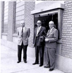
Figure 3: 1956: Walk-Up Teller Window retrofitted into existing glass block opening
