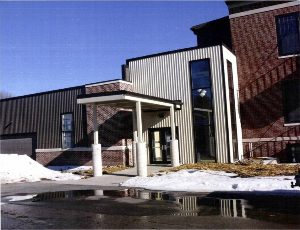
Attachment D – Atrium as Constructed (West and East Sides)
