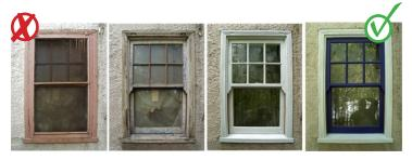
A simple process of paint restoration and repair of dry-rot and broken glass can greatly enhance the visual aesthetics of an aging building.
