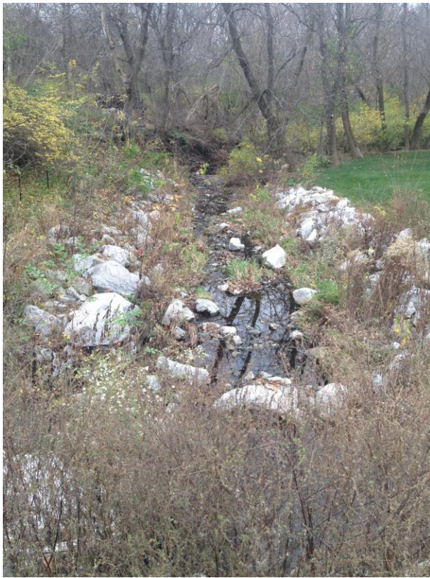
Outlet of culvert downstream of Hoover Avenue/Edgewater Drive.
