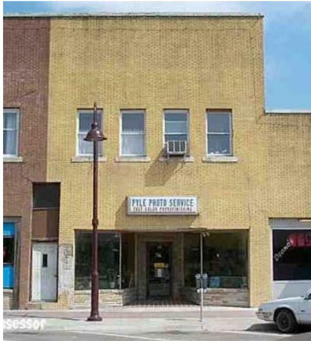
Façade at 121 Main Street before reconstruction
