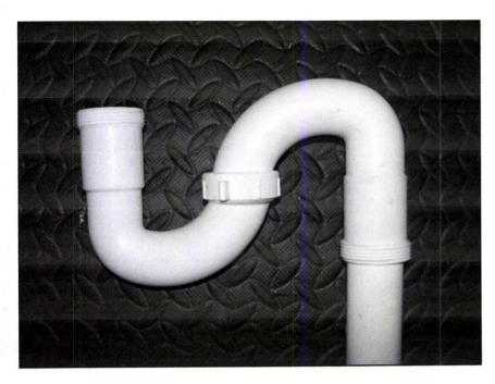
The most common places you'll find "S" traps are at plumbing fixtures that aren't vented, such as an illegal basement bathroom sink, a DIY basement bar sink, or a kitchen sink where the old steel drain in the wall was so corroded and blocked that someone installed a new drain, but never bothered to vent it.
